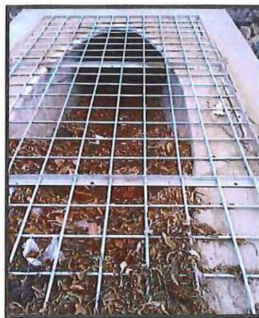
**Installed 60-inch connection pipe into Basin 8
